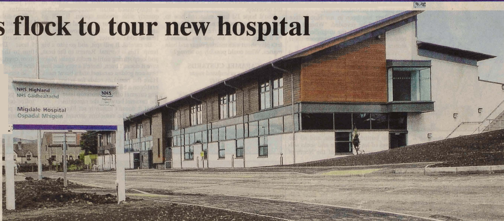
Patients and staff move into the new hospital in three weeks' time.
