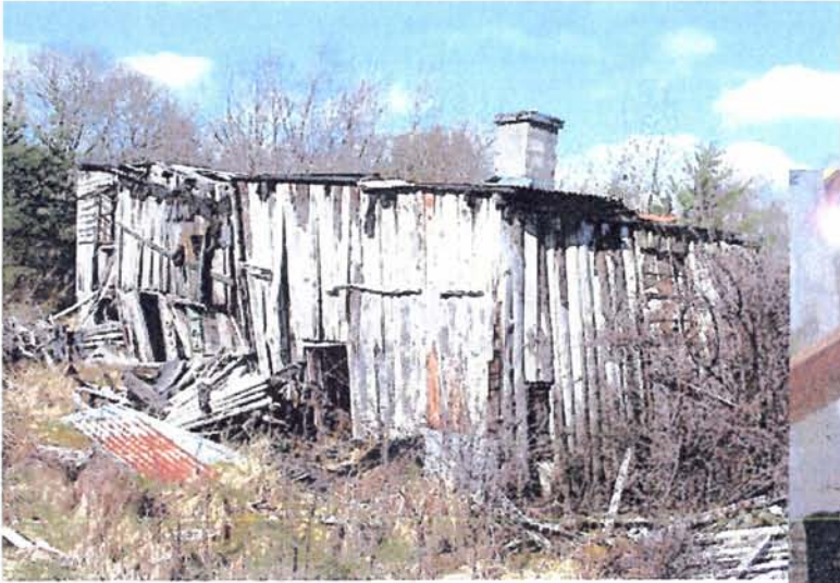
The accommodation block is still standing, but looks very unstable.
