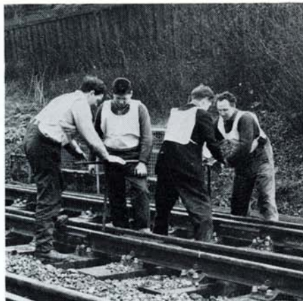
The Scottish Region has issued 15 platelayers working on the Pollokshields-Eglinton Street section of the Glasgow suburban electric line with a new kind of luminous safety jacket which shines in half-light conditions. These jackets are made from a fluorescent orange plastic material and are similar in appearance to old-fashioned ships' life-jackets.
